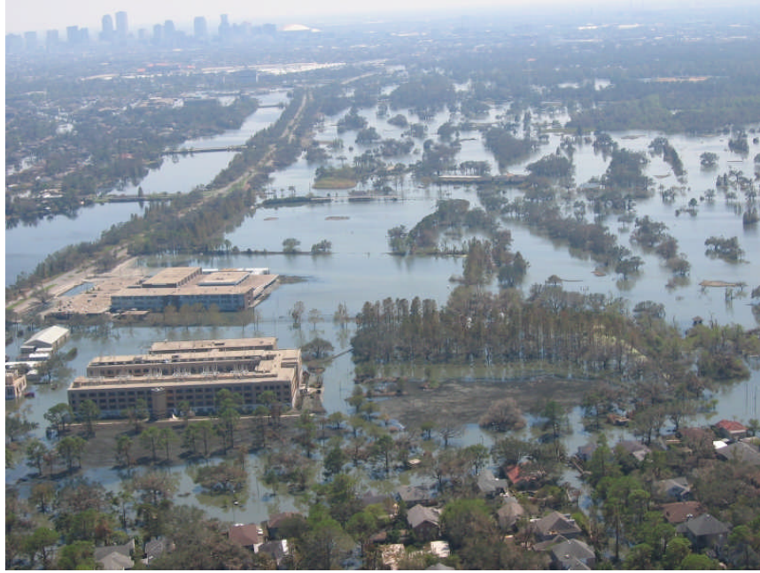
(Photo of flooded residential area after Katrina, courtesy of the National Oceanic and Atmospheric Administration)
